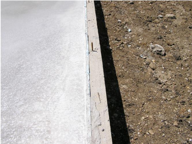
**Photograph 4: Thermal Break**—A thermal break worthy of great artisans. Install a strip of waterproofing set in mastic that spans the rigid edge insulation that acts as both a capillary break and an insect barrier.
