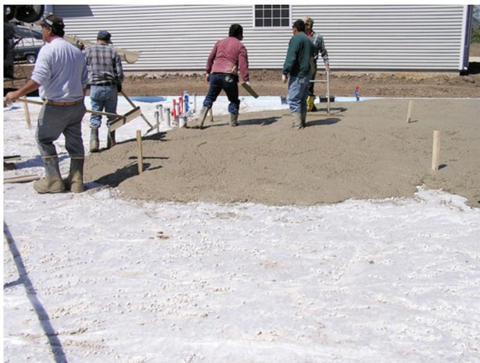
**Photograph 3: Concrete Placement**—Shows concrete being placed on the top of the sheet polyethylene and a layer of XPS insulation. Notice that there is no welded-wire mesh. Stones – gravel keep the plastic from blowing away.
