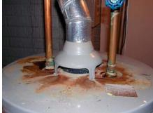
Clothes dryers, bath fans, and range hoods exhaust air from a house. If makeup air isn't supplied with a duct, it will leak in through cracks. Even worse, makeup air will be backdrafted through combustion appliances, which can cause carbonmonoxide poisoning. Using sealed-combustion appliances and makeup-air units for large range hoods gets around this problem.
